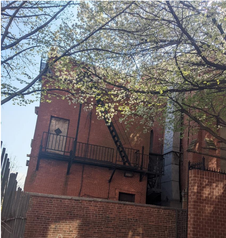
Image 5: Oblique view of the east and north elevations of the parsonage. (4/7/2021)
