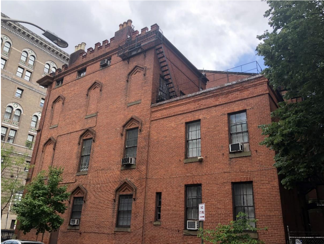
Image 4: View of the north elevation of the parsonage, facing W. Hamilton Street; image provided by applicant.
