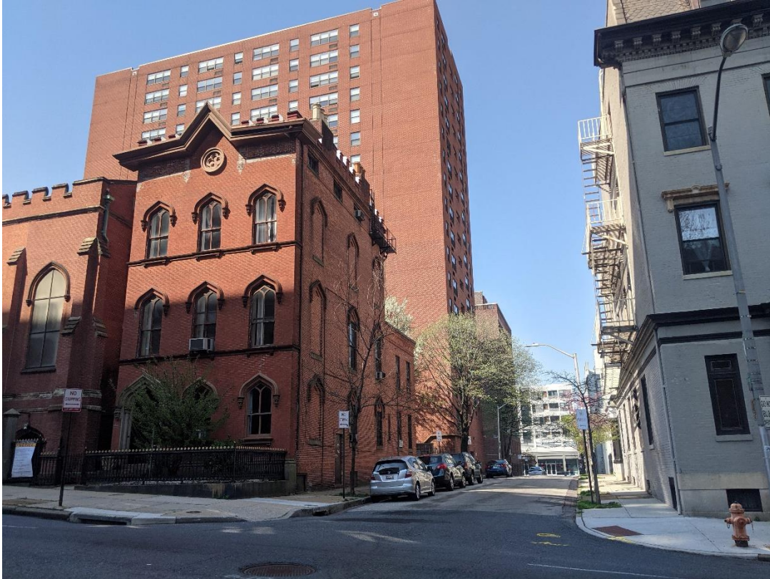
Image 2: Oblique view of the east and north elevations of the parsonage. (4/7/2021)
