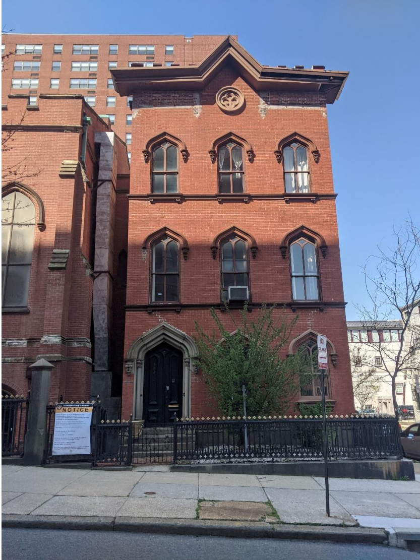
Image 1: Façade of parsonage, facing east on Cathedral Street. (4/7/2021)
