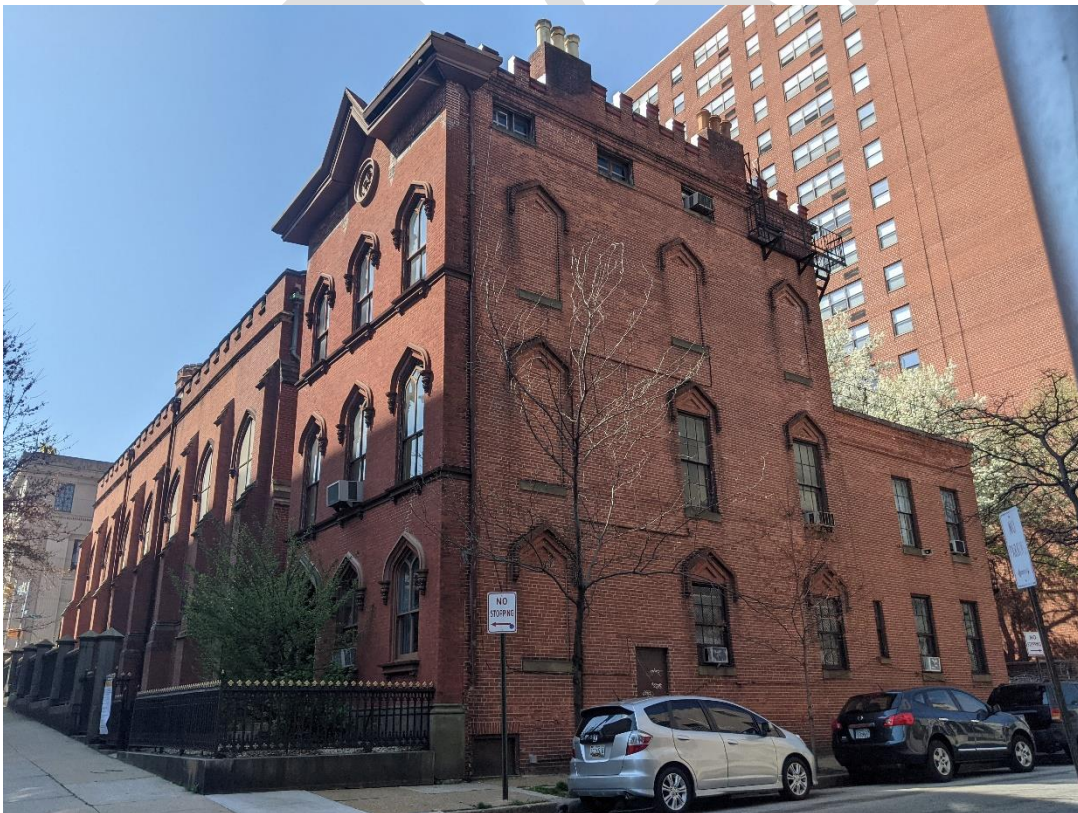
Image 3: Oblique view of the east and north elevations of the parsonage. (4/7/2021)
